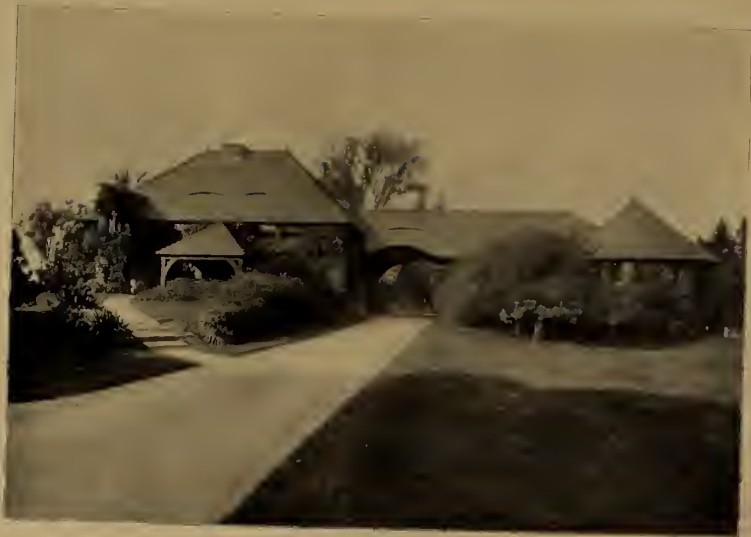
GATE LODGE AT LANGWATER. ESTATE OF MRS. FREDERICK L. AMES, North Easton, Mass.
